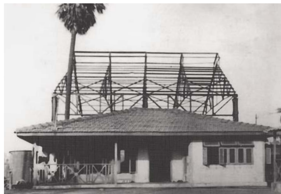
The old Excel canteen, above. "The Excel canteen is something that makes Excel stand apart," says Dr Milind Gokhale. A common canteen for workers and officers was the heart of every Excel plant and office. The canteens at Roha, Lote and Dhordo.
