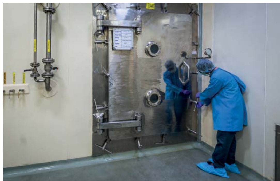
The state-of-the-art-pharma facility at Lote-Parshuram.
