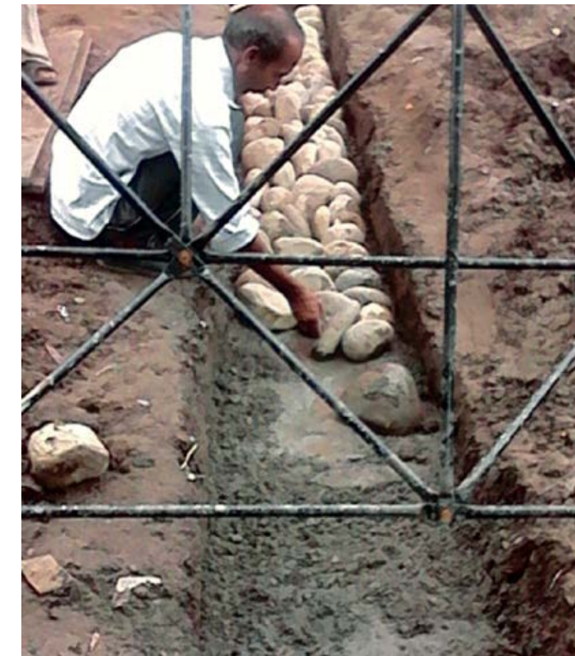
A toilet block under construction. Drawing on the local designs developed at Agrocel which enable quick assemblage, her team focused on building toilet blocks under the Swachh Bharat Abhiyan.
