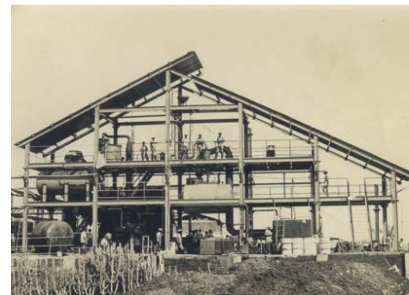
In 1975, completion of the PCI3 plant at Roha in 100 days.
