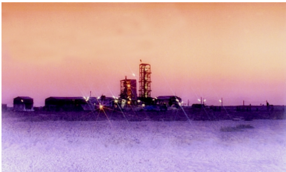
The Bromine Plant – the dream project now an actuality.
