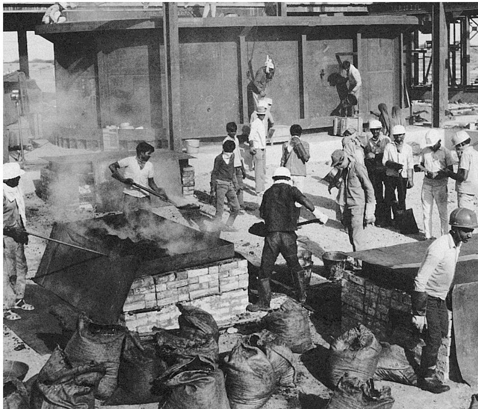
Carbon paste being poured into trays. Hazardous and tedious work that would help build the furnace.
