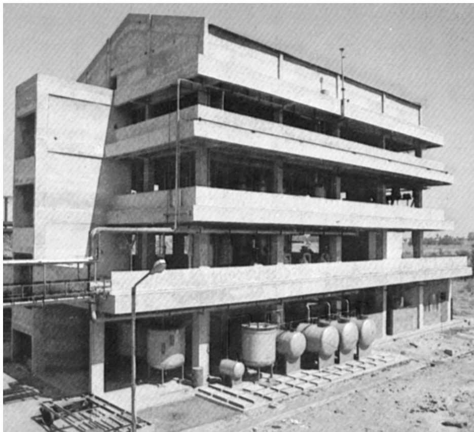
Oxalic Acid plant under construction.
