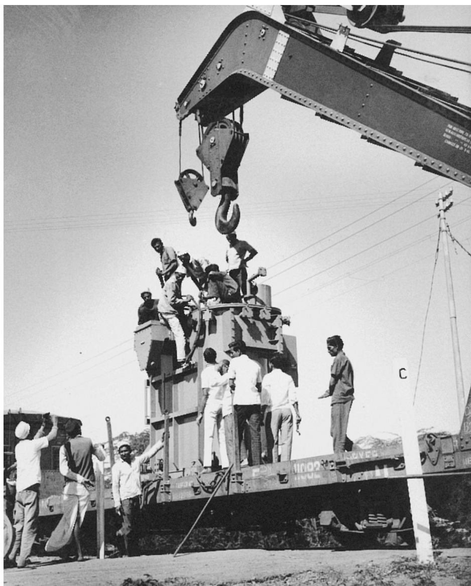
The transformer was transported by train on the Ruwapari track and the ONGC crane helped transport it to the Excel plant site at Bhavnagar.
