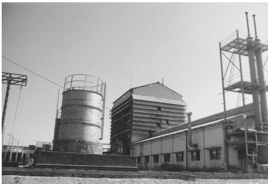
The SPCP plant at Lote Parashuram. The first plant to be commissioned at the Lote site in 1985.
