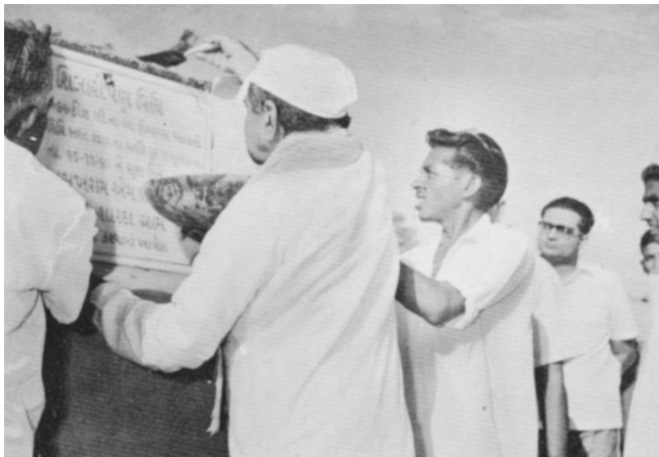
Mansukhram Jobanputra laying the foundation stone of the Phosphorus project in November 1969.
