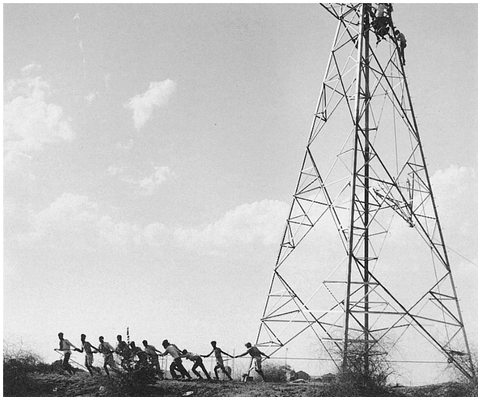
Assembling the transmission line tower for Excel. "A Herculean task for all the obstacles that came our way . . ." in the words of Kaka. The team-spirit is what made the difference!
