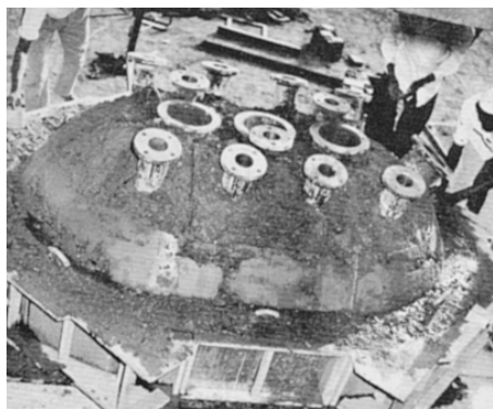
Phosphorus furnace roof as seen from the top.
