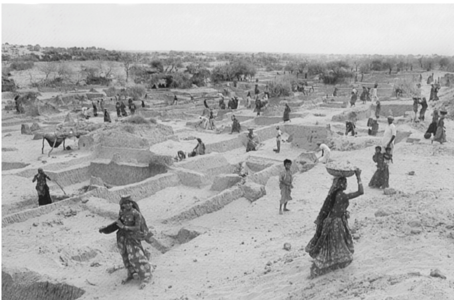
Digging a tank for relief work during drought in Kutch.
