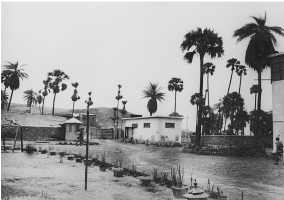
Amboli site being developed with a proper boundary wall and entrance gate.
